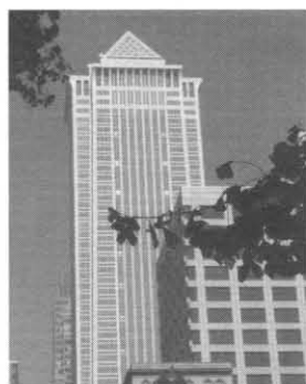
The Pyramid Club atop the Mellon Bank Building - site of the AGLP Opening Reception
