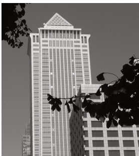
The Pyramid Club atop the Mellon Bank Building - site of the AGLP Opening Reception
