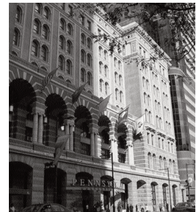
The new Pennsylvania Convention Center was created from the original Reading Company train shed and headhouse.
